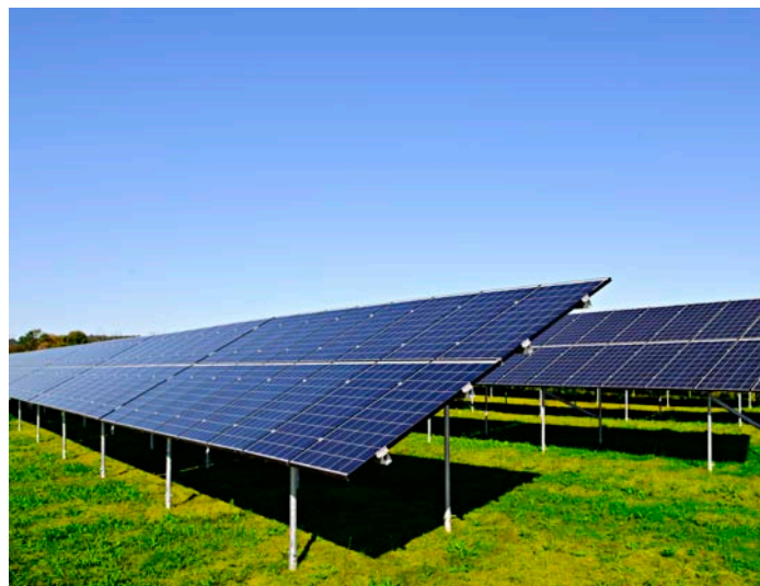
Fig. 3 A system after cleaning.
