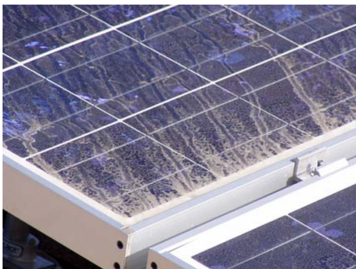
Fig. 2 Dust fall on solar panels.
